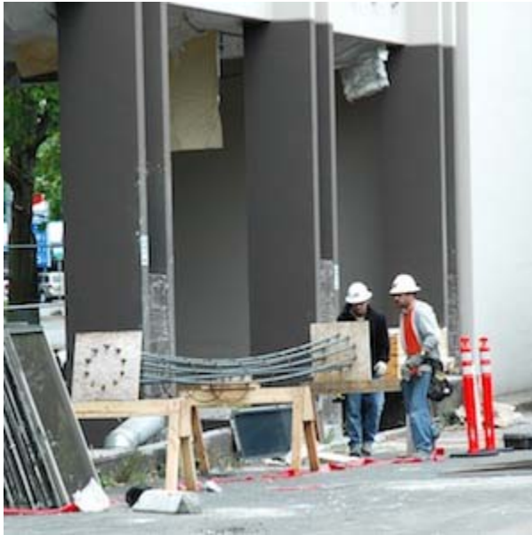
Workers prepare to reinforce non-ductile columns.
